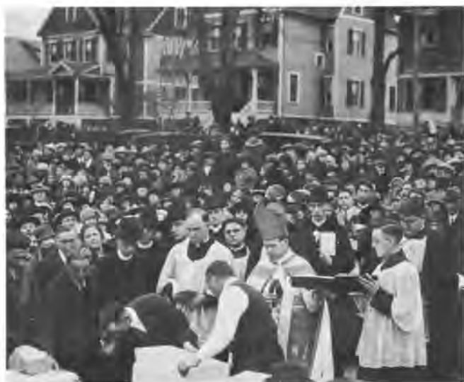
Laying of the Cornerstone and breaking ground for Sacred Heart Church.
